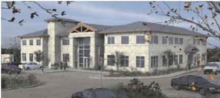
TxDOT administration building where customer service and violation processing operations are located.
