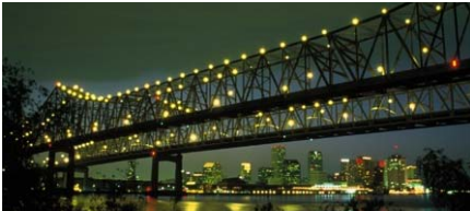
The Crescent City Connection bridge in New Orleans.
