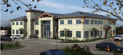
TxDOT administration building where customer service and violation processing operations are located.
